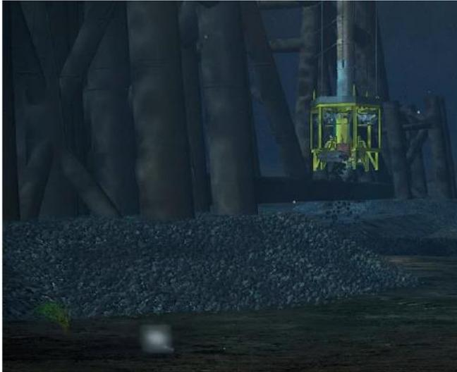
Fig 2 – Example of rock being placed via fall pipe end and ROV
